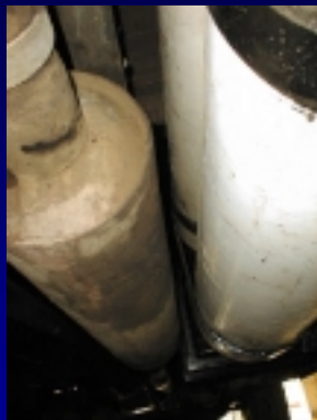
CNG cylinder next to exhaust
