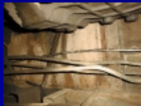
No stress loops / piping too rigid / unsupported piping
